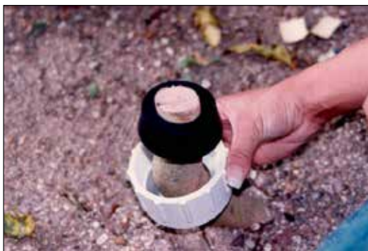
Photo 10 Installing the compression ring
